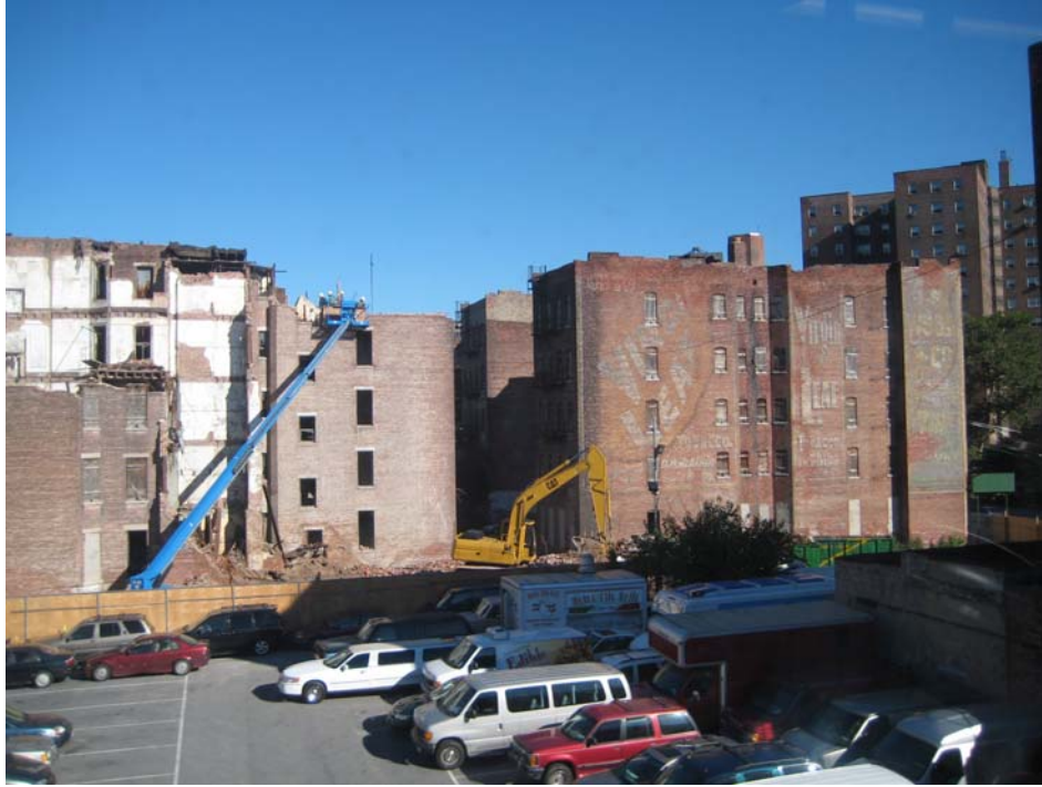
Vacant Housing in Secondary Study Area West of Park Avenue Under Demolition in 2007
